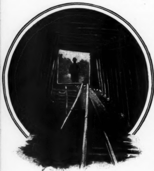
LOOKING UP THE MAN WAY TOWARD THE SURFACE.
